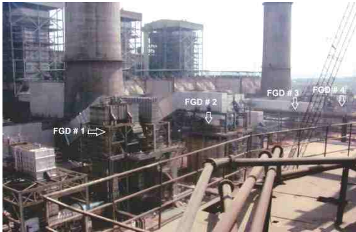
Aerial View of all 4 FGD Units
